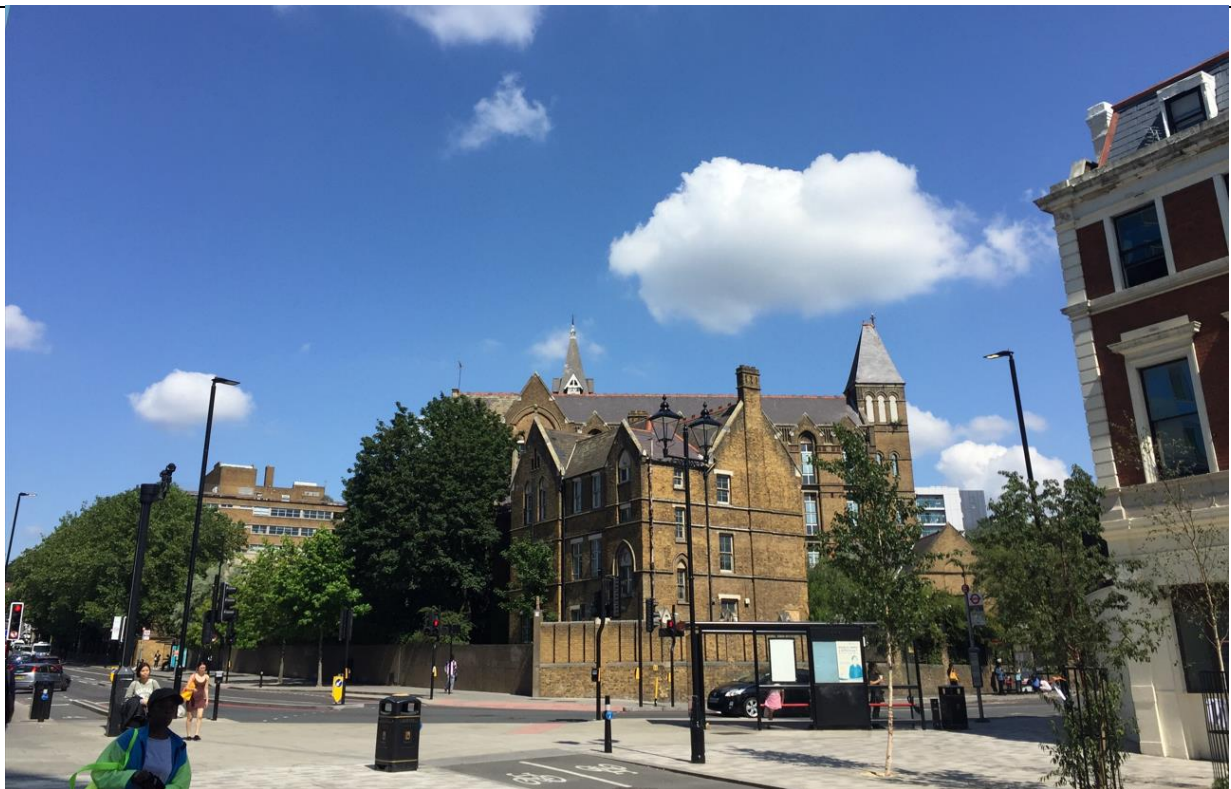
Figure 5: Southern apex of the site and nurses wing looking north east from Navigator Square
