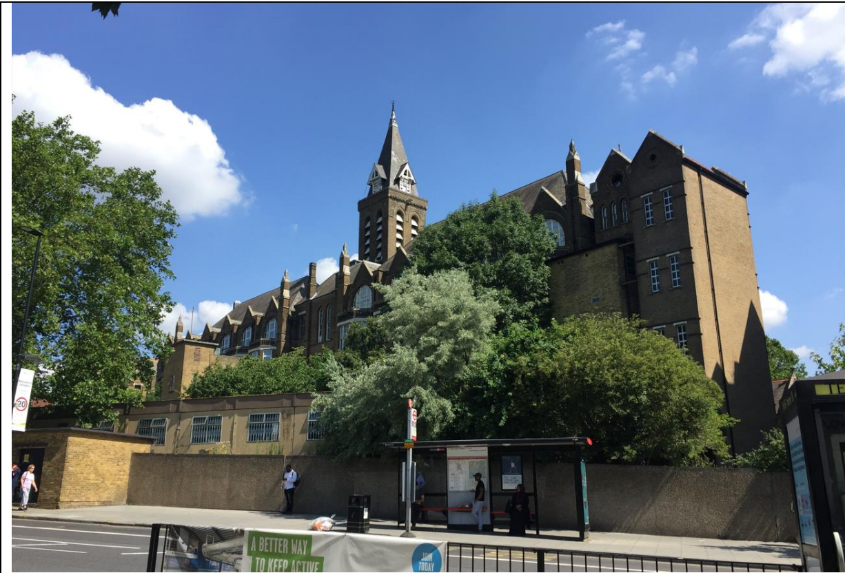
Figure 6: Western (rear) elevation of the Holborn Union Main Range building, looking north east from Highgate Hill
