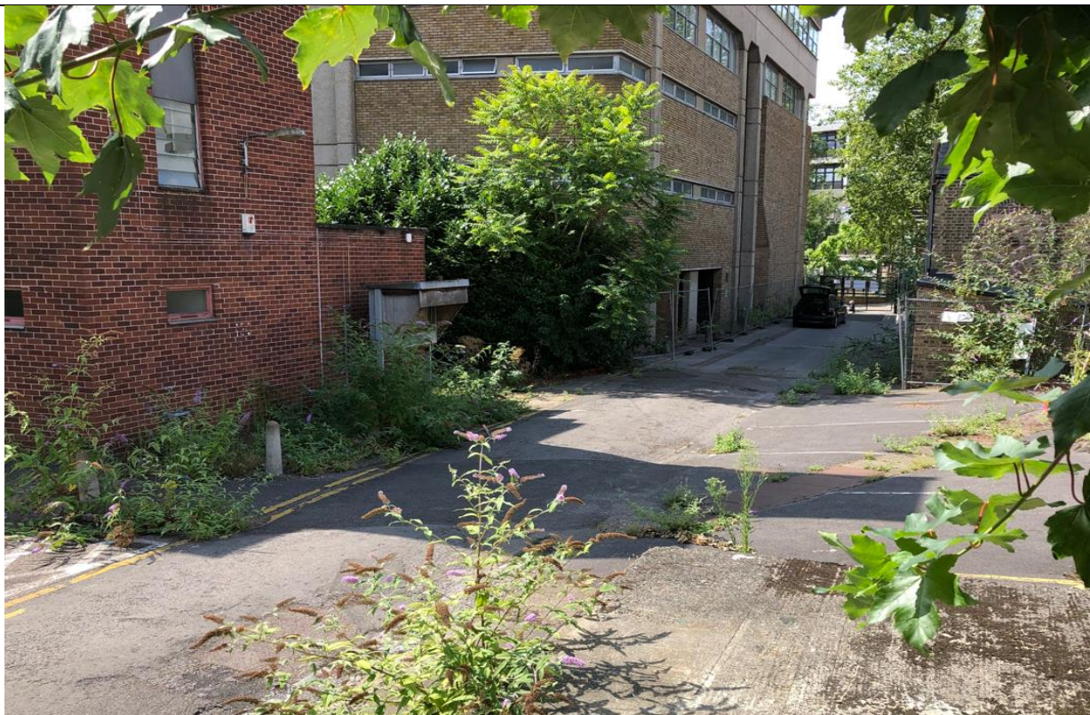
Figure 11: Northern elevations of the Ely building (left) and Furnival building (right) and access road across the northern part of the site – looking west from the northern boundary of the site
