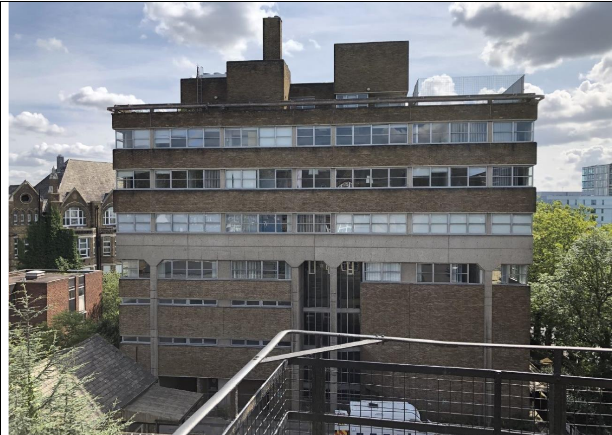
Figure 10: The Furnival building, looking south from The Academy (neighbouring residential building)
