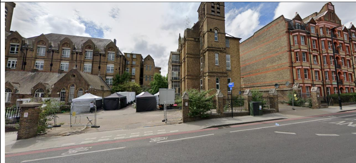
Figure 13: Existing vehicular access points to the site from Archway Road
